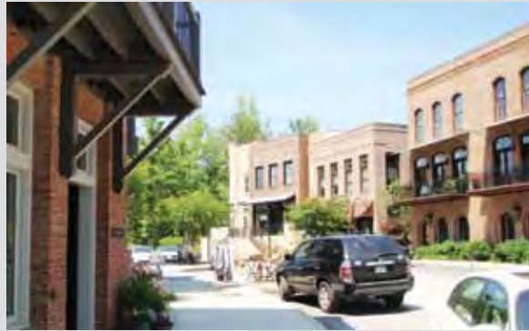
Photo 4.39 Mixed-use buildings, Serenbe, GA
