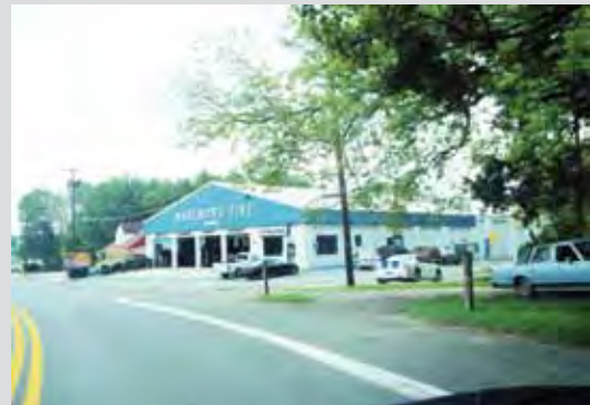
Photo 2.13: MD 725/Marlboro Pike—Looking East
