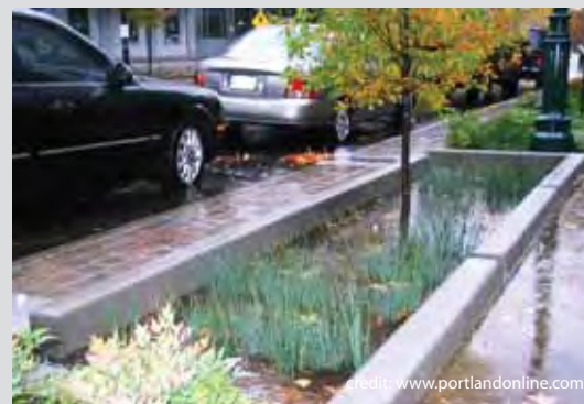
Photo 4.9 Rainwater Planter, Portland, OR
