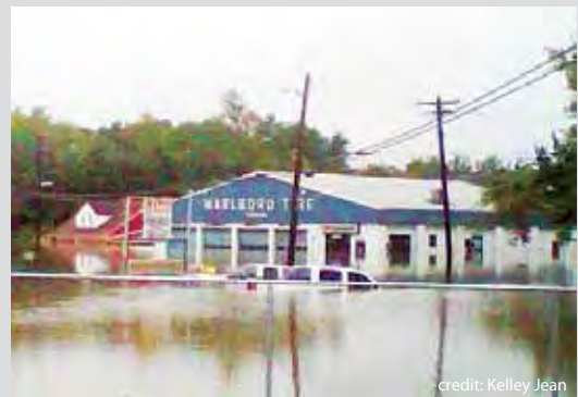
Photo 2.2 MD 725/Marlboro Pike after Flooding
