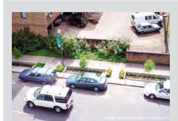
Photo 4.6 Rainwater Planter, Portland, OR
