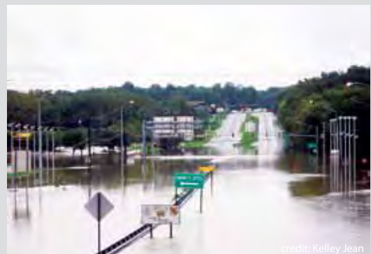
Photo 2.3 US 301/Crain Hwy.—High Water after Flooding
