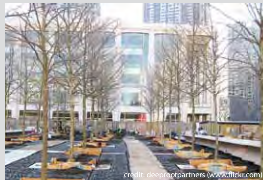
Photo 4.12 Silva Cell Construction, Lincoln Center, NY, NY
